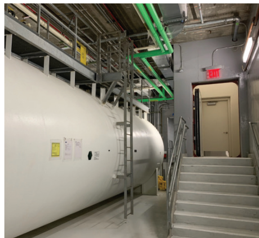
The David H. Koch Center for Cancer Care’s property line and exterior walls were reinforced and waterproofed with floodgate technology to withstand storm surges, and part of its infrastructure includes a submarine-style waterproof entry door to the fuel tank room which serves its heating plant and emergency power systems.
